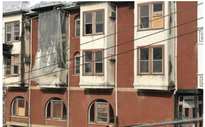
BEFORE: The Flat Iron Building
